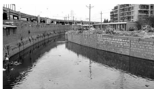
入滇河道寬槽河整治前
